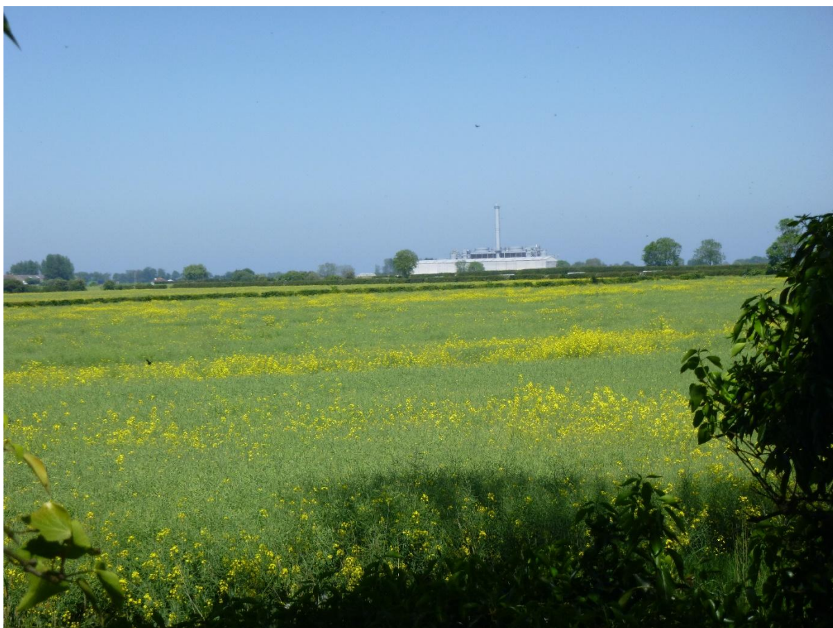
The Biomass Power Plant
